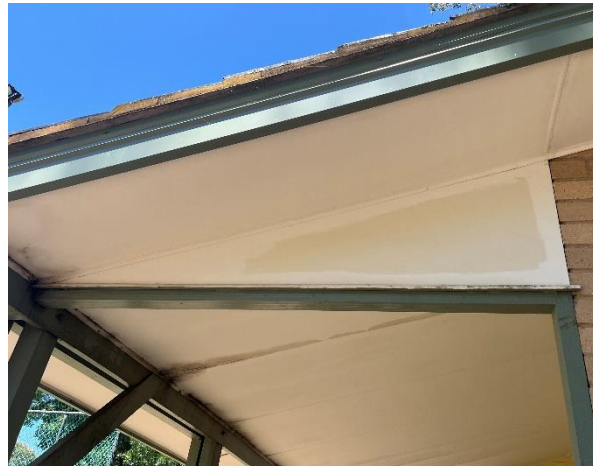
Line ID 22: External, Building 19 Lodges 5-8, Perimeter Verandas, Eave Lining, Fibre Cement Sheet - Chrysotile Asbestos Detected
