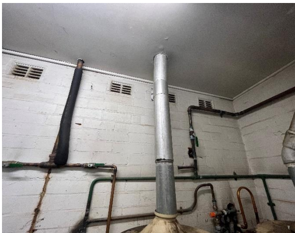
Line ID 62: Internal, Building 21 Ablutions Block, Boiler Room, Flue Pipes, Moulded Fibre Cement Pipes - Chrysotile & Amosite Asbestos Detected
