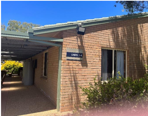
Line ID 19: External, Building 18 Lodges 1-4, Perimeter Verandas, Gable Ends Tile Support Strips, Fibre Cement Sheet - Chrysotile Asbestos Detected
