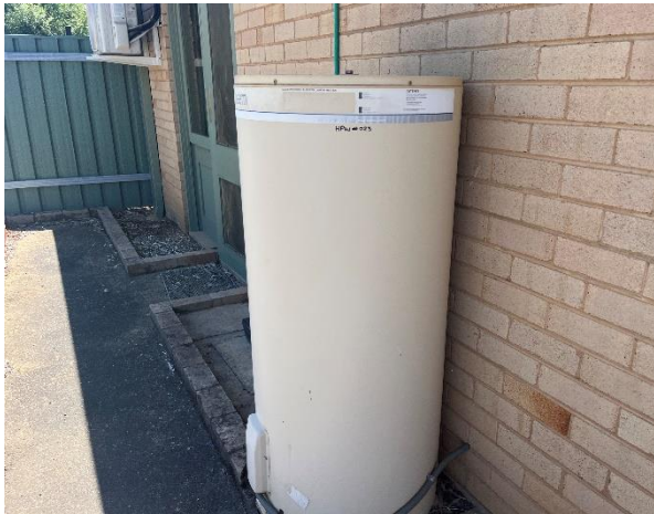
Line ID 85: External, Residence 16, Entry Area and Surrounds, Hot Water Unit, Insulation Material - Suspected SMF
