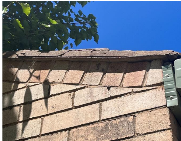
Line ID 3: External, Building 10 General Managers Office, Perimeter Verandas, Gable End Tile Support Strips, Fibre Cement Sheet - Chrysotile Asbestos Detected
