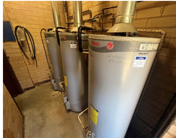
Line ID 94: Internal, Building 26 & 27 Kitchen & Dining Room, Boiler Room, Hot Water Units, Insulation Material - Suspected SMF
