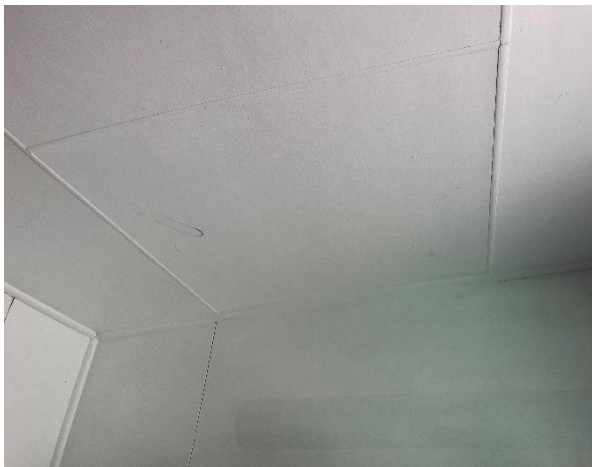
Line ID 73: Internal, Craft Shed, Bush craft and Sports Store, Ceiling and Wall Linings, Fibre Cement Sheet - Chrysotile Asbestos Detected
