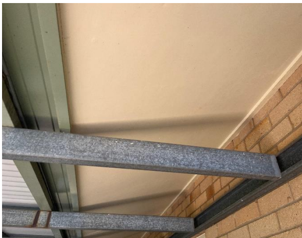
Line ID 25: External, Building 20 Lodges 9-12, Perimeter Verandas, Eave Lining, Fibre Cement Sheet - Chrysotile Asbestos Detected
