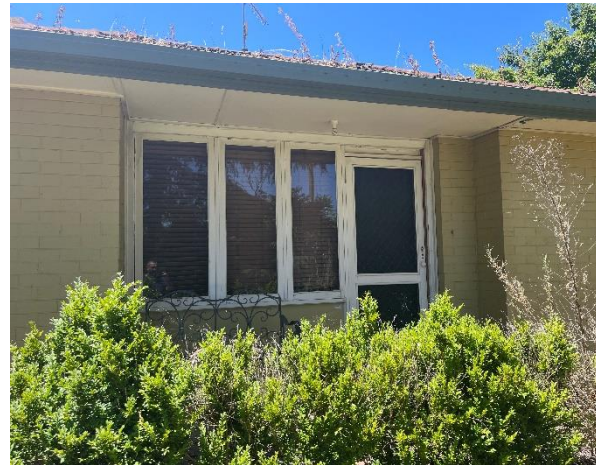
Line ID 12: External, Building 12 Client Services Coordinator Residence, Perimeter Verandas, Bathroom & Kitchen Wall Lining, Fibre Cement Sheet - Chrysotile Asbestos Detected
