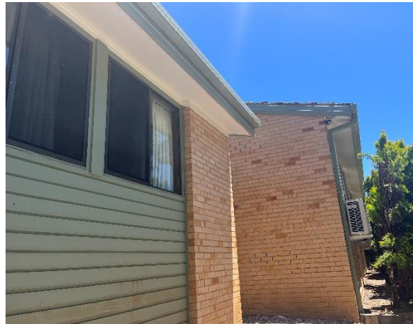
Line ID 28: External, Building 21 Ablutions Block, Entry and Covered Walkway Area, Eave Lining, Fibre Cement Sheet - Chrysotile Asbestos Detected
