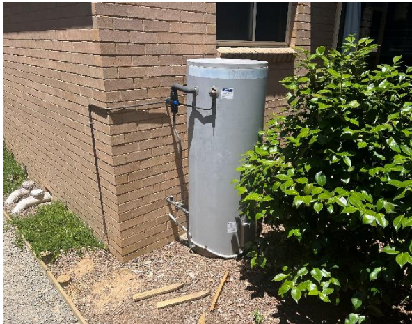
Line ID 81: External, Building 18 Lodges 1-4, Perimeter Verandas, Hot Water Units, Insulation Material - Suspected SMF
