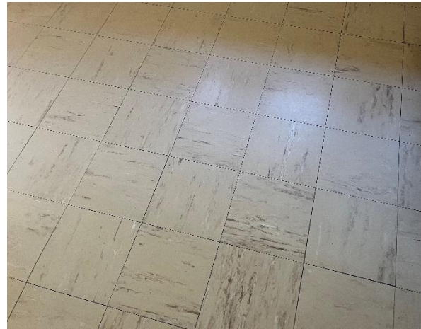
Line ID 72: Internal, Building 26 & 27 Kitchen & Dining Room, Staff Area, Throughout the Kitchen Staff Area, Beige Vinyl Floor Tiles - Chrysotile Asbestos Detected
