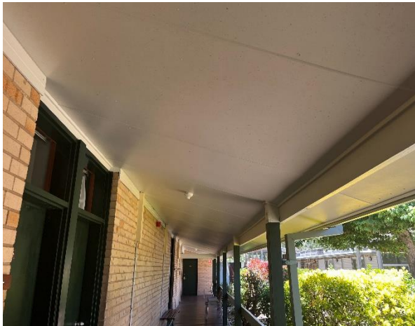
Line ID 27: External, Building 21 Ablutions Block, Entry and Covered Walkway Area, Ceiling Lining to Internal & External Verandas, Fibre Cement Sheet - Chrysotile Asbestos Detected
