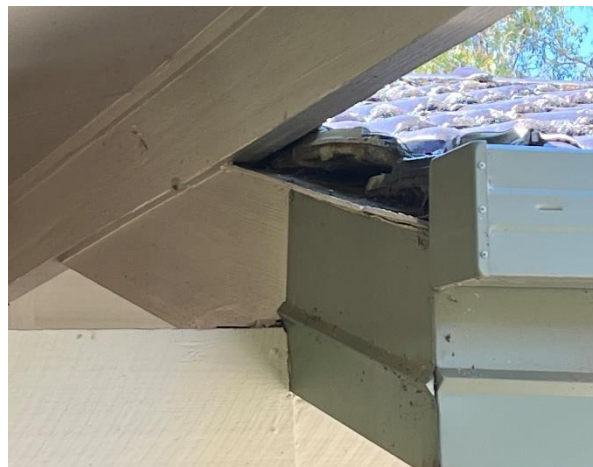
Line ID 26: External, Building 20 Lodges 9-12, Perimeter Verandas, Gable Ends Tile Support Strips, Fibre Cement Sheet - Chrysotile Asbestos Detected
