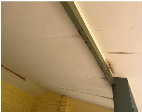
Line ID 50: External, Tennis Club House, Kitchen and Covered Area, Awning Lining, Fibre Cement Sheet - Chrysotile Asbestos Detected
