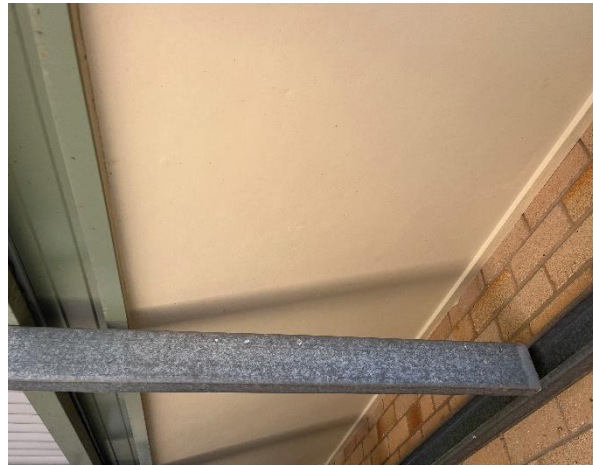
Line ID 18: External, Building 18 Lodges 1-4, Perimeter Verandas, Eave Lining, Fibre Cement Sheet - Chrysotile Asbestos Detected
