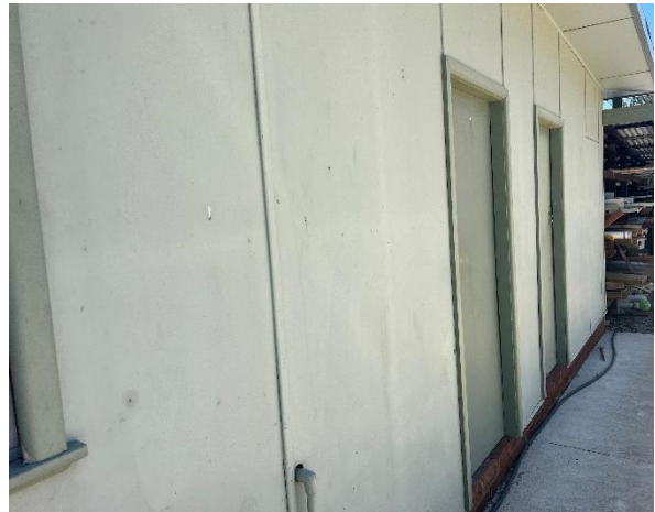
Line ID 42.1: External, Maintenance Garage, Garage, West Wall Cladding, Fibre Cement Sheet - Chrysotile Asbestos Detected
