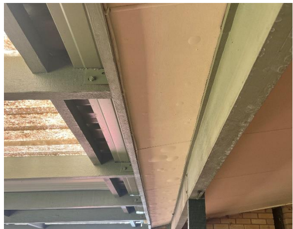
Line ID 6: External, Building 11 Service Coordinator Residence, Perimeter Verandas, Eaves, Fibre Cement Sheet - Chrysotile Asbestos Detected
