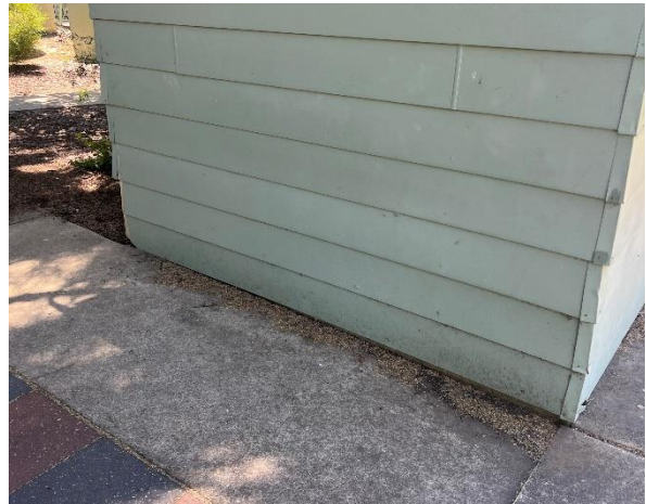
Line ID 38: External, Craft Shed, Perimeter Areas, Wall Cladding to All Sides, Fibre Cement Sheet - Chrysotile Asbestos Detected
