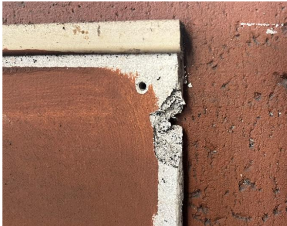
Line ID 77: Internal, Maintenance Workshop Metal, Workshop, To Wall Behind Work Bench, Fibre Cement Sheet - Chrysotile Asbestos Detected
