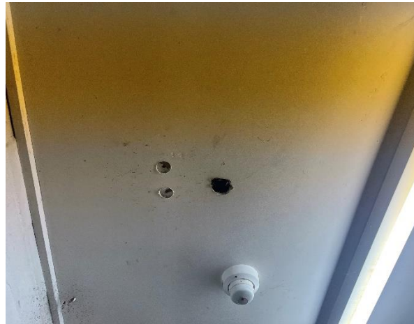
Line ID 61.1: Internal, Building 21 Ablutions Block, Boiler Room, Ceiling Lining to the Boiler and Cleaners Room, Fibre Cement Sheet - Chrysotile Asbestos Detected
