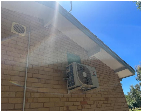
Line ID 29: External, Building 21 Ablutions Block, Entry & Covered Walkway Area, Gable Ends, Fibre Cement Sheet - Chrysotile Asbestos Detected
