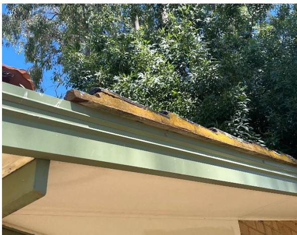
Line ID 53: External, Tennis Club House, Kitchen and Covered Area, Gabled Roof Ends Tile Edge Support, Fibre Cement Sheet - Chrysotile Asbestos Detected
