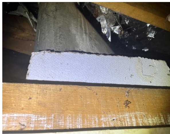
Line ID 63: Internal, Building 21 Ablutions Block, Boiler Room, Packer Within the Ceiling to the Hatch, Fibre Cement Sheet Packer - Chrysotile Asbestos Detected
