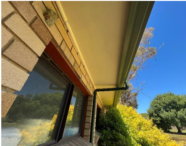
Line ID 76: Internal, Cricket Club House, Veranda, Eaves, Fibre Cement Sheet - Chrysotile Asbestos Detected
