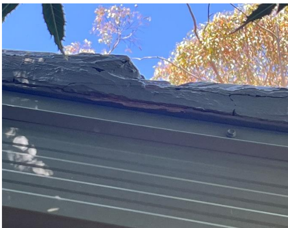
Line ID 40: External, Cricket Club House, Roof, Gable Ends of the Roof Tile Supports, Fibre Cement Sheet - Chrysotile Asbestos Detected
