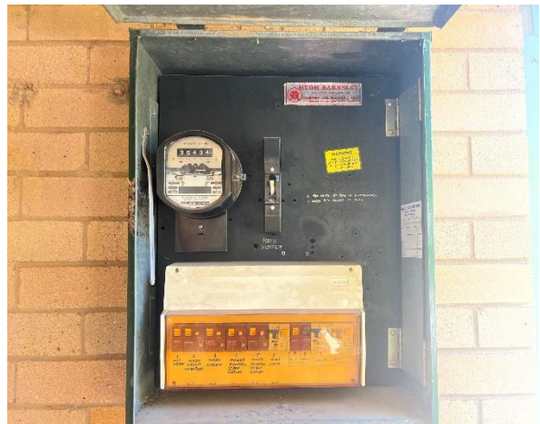
Line ID 47: External, Residence 16, Entry Area and Surrounds, Southside Electrical Box, Bituminous Backing Board - Chrysotile Asbestos Detected
