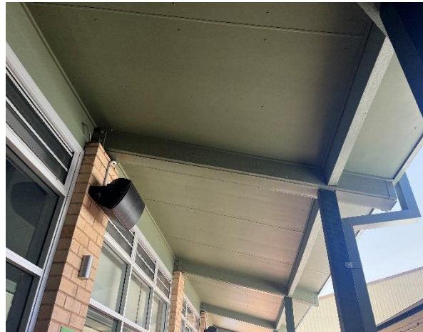
Line ID 32: External, Building 26 & 27 Kitchen, Entry and Covered Walkways, Eaves, Fibre Cement Sheet - No Asbestos Detected
