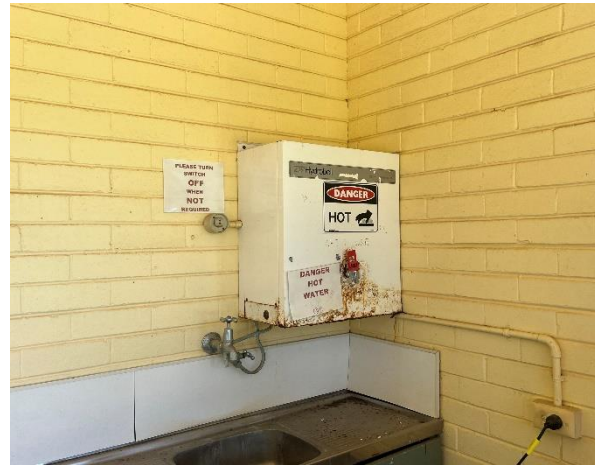
Line ID 86: External, Tennis Club House, Kitchen and Covered Area, Hot Water Unit, Insulation Material - Suspected SMF
