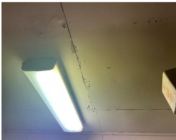
Line ID 78: Internal, Site 17 Maintenance Workshop Wood, Workshop and Office, Ceiling Lining, Fibre Cement Sheet - Chrysotile Asbestos Detected
