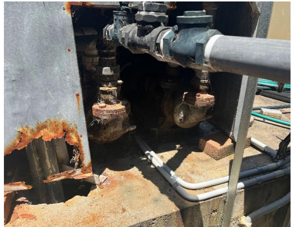
Line ID 49: External, Site 17 Maintenance Workshop Wood, Entry Area, Adjacent the Garage, Water Pump Pipework Gaskets, Gasket Material - Chrysotile Asbestos Detected
