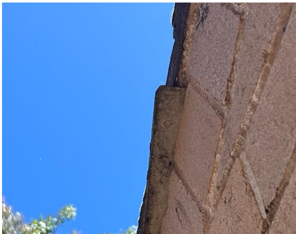
Line ID 46: External, Residence 16, Entry Area and Surrounds, Gable Ends Tile Support Strip, Fibre Cement Sheet - Chrysotile Asbestos Detected
