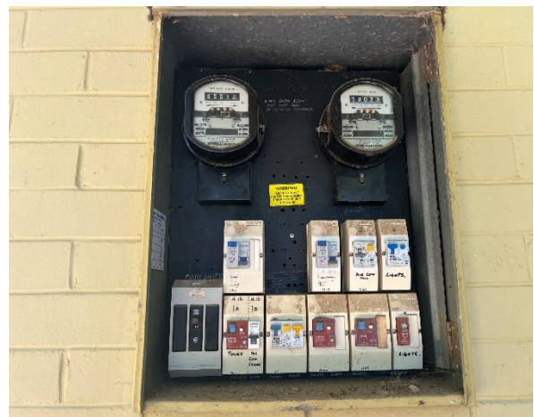
Line ID 15: External, Building 12 Client Services Coordinator Residence, Perimeter Verandas, South Side Electrical Box, Bituminous Backing Board - Chrysotile Asbestos Detected
