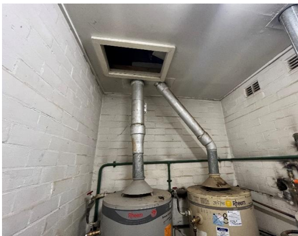
Line ID 62.2: Internal, Building 21 Ablutions Block, Boiler Room, Flue Pipes to Hot Water Units, Moulded Fibre Cement Pipes - Chrysotile & Amosite Asbestos Detected
