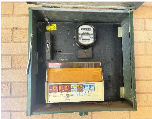
Line ID 4: External, Building 10 General Managers Office, Perimeter Verandas, South Side Electrical Box, Bituminous Backing Board - Chrysotile Asbestos Detected
