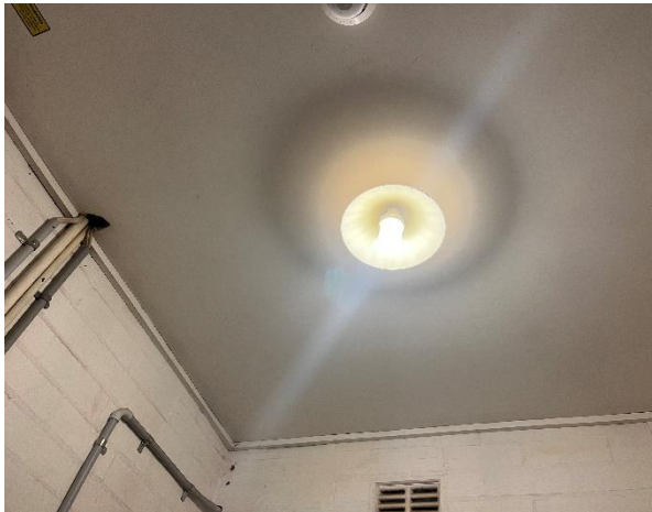
Line ID 61: Internal, Building 21 Ablutions Block, Boiler Room, Ceiling Lining to the Boiler and Cleaners Room, Fibre Cement Sheet - Chrysotile Asbestos Detected
