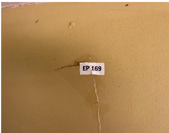
Line ID 14.1: External, Building 12 Client Services Coordinator Residence, Perimeter Verandas, Garage Wall Lining, Fibre Cement Sheet - Chrysotile Asbestos Detected
