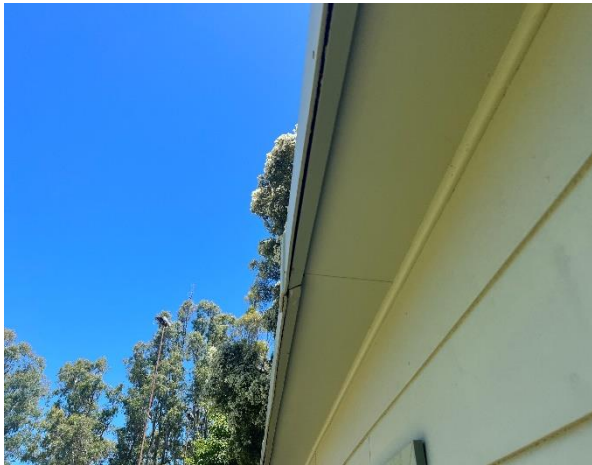
Line ID 36: External, Craft Shed, Perimeter Areas, Eaves, Fibre Cement Sheet - Chrysotile Asbestos Detected
