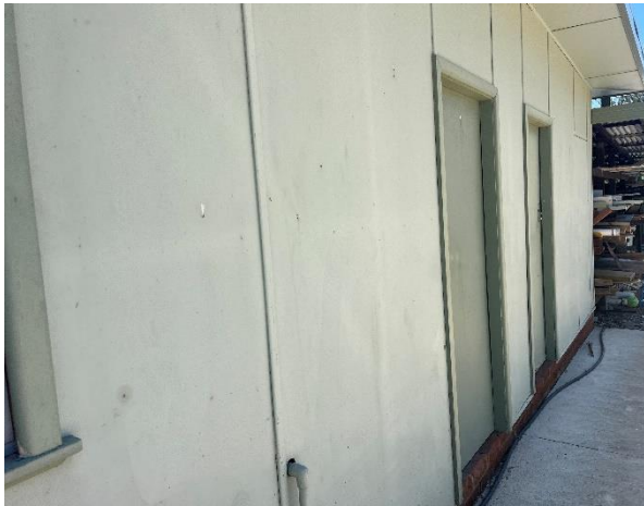
Line ID 48: External, Site 17 Maintenance Workshop Wood, Entry Area, Wall Cladding & Eaves, Fibre Cement Sheet - Chrysotile Asbestos Detected
