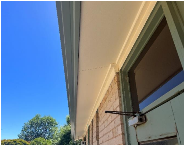
Line ID 2: External, Building 10 General Managers Office, Perimeter Verandas, Eaves, Fibre Cement Sheet - Chrysotile Asbestos Detected
