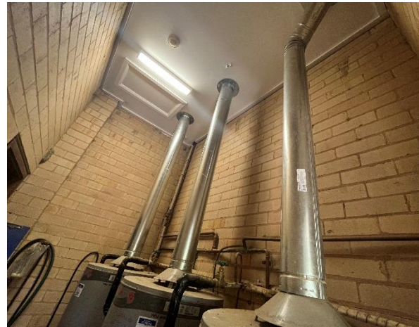
Line ID 65: Internal, Building 26 & 27 Kitchen & Dining Room, Boiler Room, to Boiler, Flue Pipes - Chrysotile Asbestos Detected
