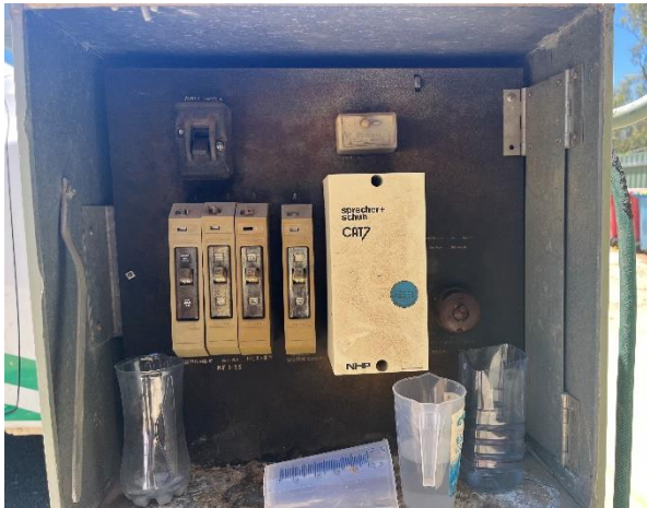
Line ID 43: External, Maintenance Workshop Metal, Externals, Adjacent Entry Roller Door, Bituminous Backing Board - Chrysotile Asbestos Detected
