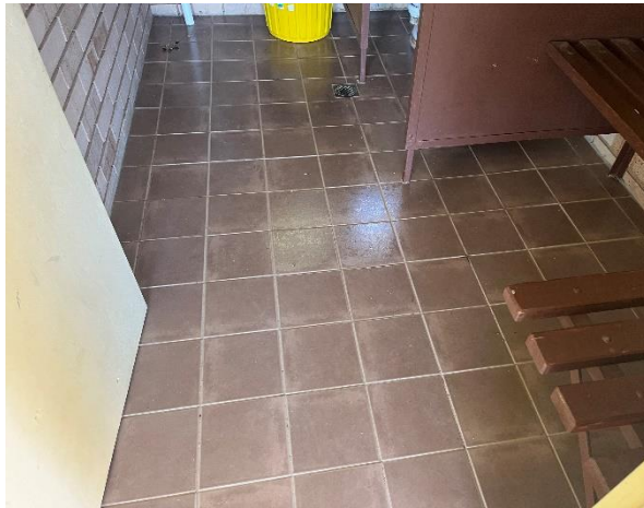
Line ID 75.1: Internal, Cricket Club House, Veranda, Below Ceramic Tiles to the Floor, Compressed Cement Sheet - Suspected Asbestos
