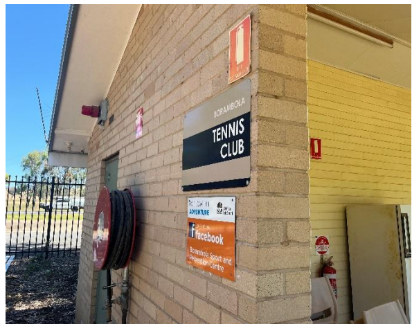
Line ID 52: External, Tennis Club House, Kitchen and Covered Area, Eaves, Fibre Cement Sheet - Chrysotile Asbestos Detected
