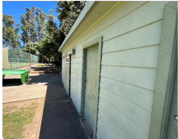
Line ID 37: External, Craft Shed, Perimeter Areas, Roof Edges and Returns, Fibre Cement Sheet - Chrysotile Asbestos Detected
