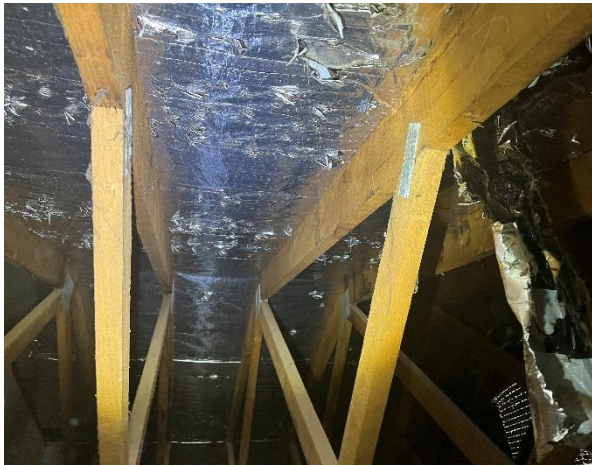
Line ID 91: Internal, Building 21 Ablutions Block, Ceiling Void, To the Underside of the Roof, Sarking Insulation - Suspected SMF
