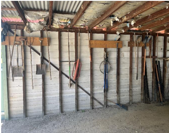
Line ID 42: External, Maintenance Garage, Garage, West Wall Cladding, Fibre Cement Sheet - Chrysotile Asbestos Detected
