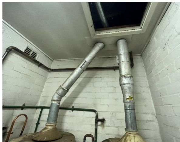
Line ID 62.1: Internal, Building 21 Ablutions Block, Boiler Room, Flue Pipes to Hot Water Units, Moulded Fibre Cement Pipes - Chrysotile & Amosite Asbestos Detected
