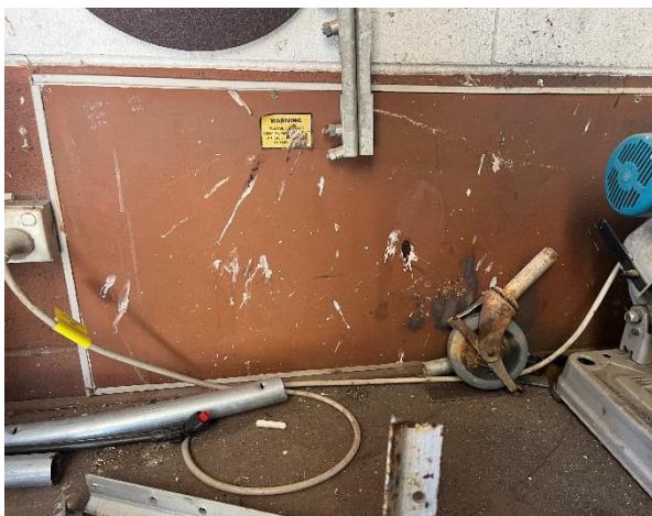
Line ID 77.1: Internal, Maintenance Workshop Metal, Workshop, To Wall Behind Work Bench, Fibre Cement Sheet - Chrysotile Asbestos Detected
