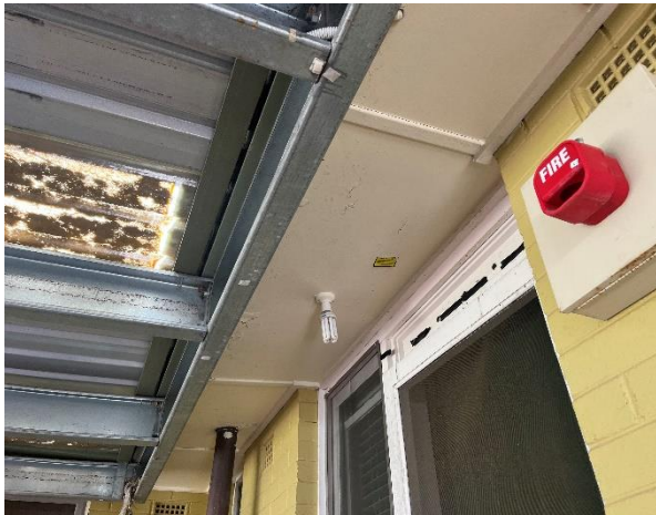
Line ID 11: External, Building 12 Client Services Coordinator Residence, Perimeter Verandas, Eaves, Fibre Cement Sheet - Chrysotile Asbestos Detected
