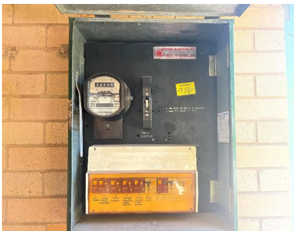
Line ID 8: External, Building 11 Service Coordinator Residence, Perimeter Verandas, Southside Electrical Box, Backing Board - Chrysotile Asbestos Detected
