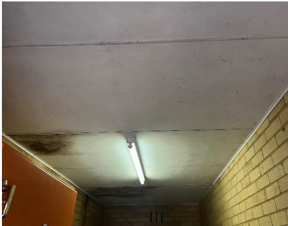
Line ID 79: Internal, Tennis Club House, Rear Electrical Cupboard, Ceiling Lining, Fibre Cement Sheet - Chrysotile Asbestos Detected
