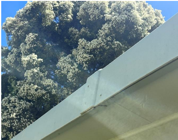
Line ID 37.1: External, Craft Shed, Perimeter Areas, Roof Edges and Returns, Fibre Cement Sheet - Chrysotile Asbestos Detected
