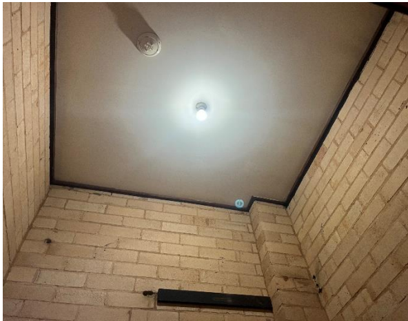
Line ID 68: Internal, Building 26 & 27 Kitchen & Dining Room, Cleaners Room, Ceiling Lining, Fibre Cement Sheet - Chrysotile Asbestos Detected
