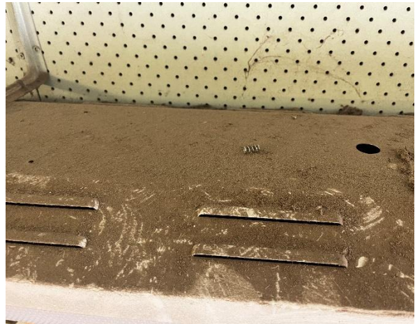
Line ID 80: Internal, Site 17 Maintenance Workshop Wood, Workshop and Office, To High level Ledges, Dust - Lead Detected (100mg/kg)
