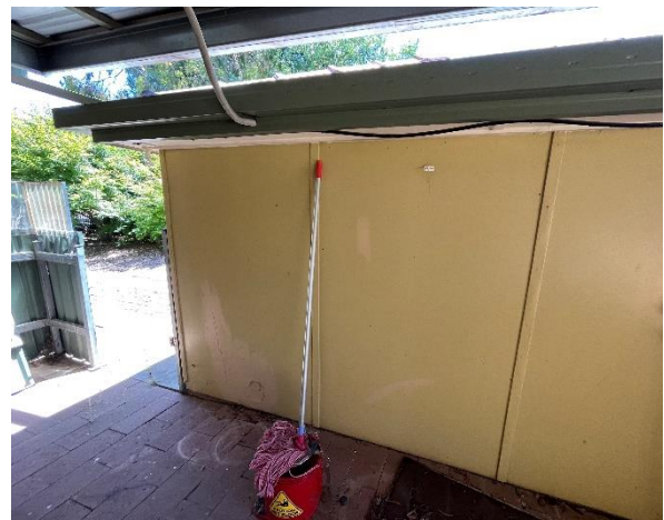
Line ID 14: External, Building 12 Client Services Coordinator Residence, Perimeter Verandas, Garage Wall Lining, Fibre Cement Sheet - Chrysotile Asbestos Detected
